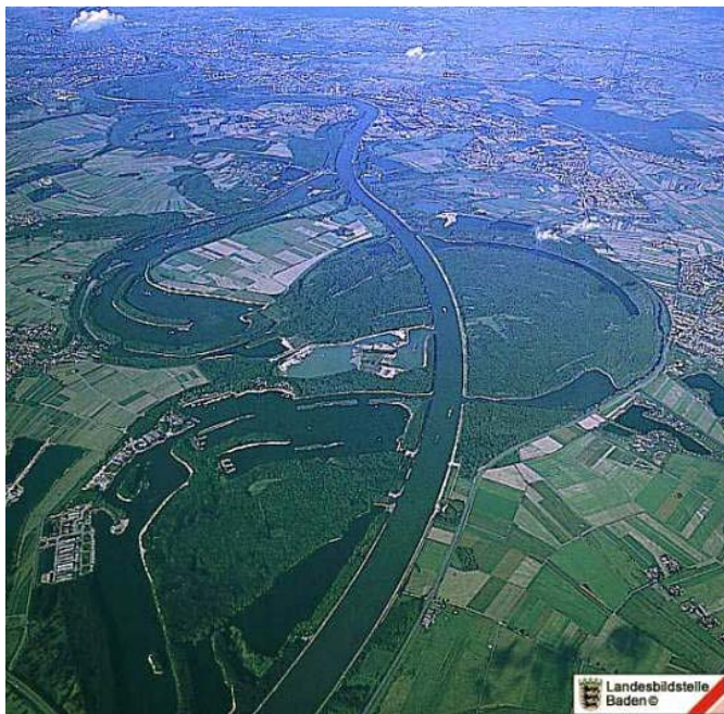
Figure 1. Rhine River at Ketsch near Heidelberg, showing large flood plains, branches and lakes, being flow effective during high flows, but ineffective during low flows (Source: Landesmedienzentrum Baden-Württemberg)
